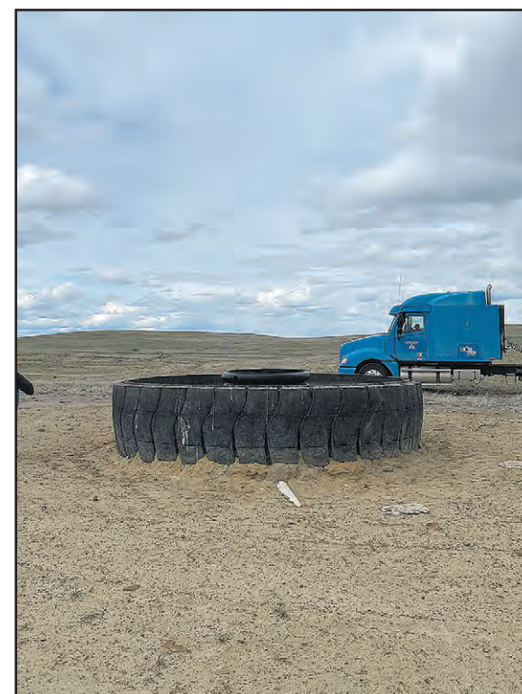
Smoothing dirt around tank in preparation for Stock Step installation.
