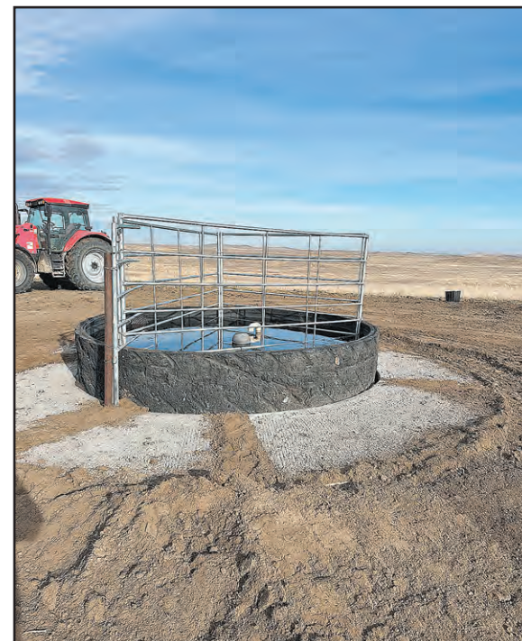
Round tank is finished with Stock Step concrete surround.
